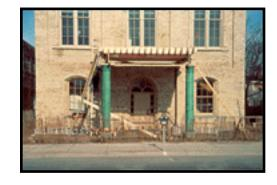
refinishing of the fancy woodwork; repair of the slate roof; the building of one chimney in place of the original four; the replacement of window-sashes; and the addition of a front portico with
