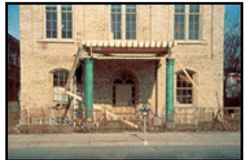
"Work on the building included light sandblasting of the bricks, which are three to five bricks thick, the interior ones completely free of salt damage; repointing of the mortar; scraping and refinishing of the fancy woodwork; repair of the slate roof; the building of one chimney in place of the original four; the replacement of window-sashes; and the addition of a front portico with
